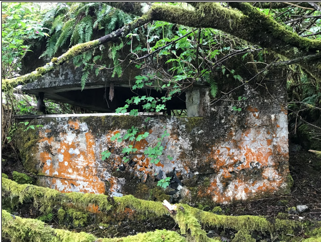
Photograph 1: Northwest Exterior of Observation Post (May 2020)
