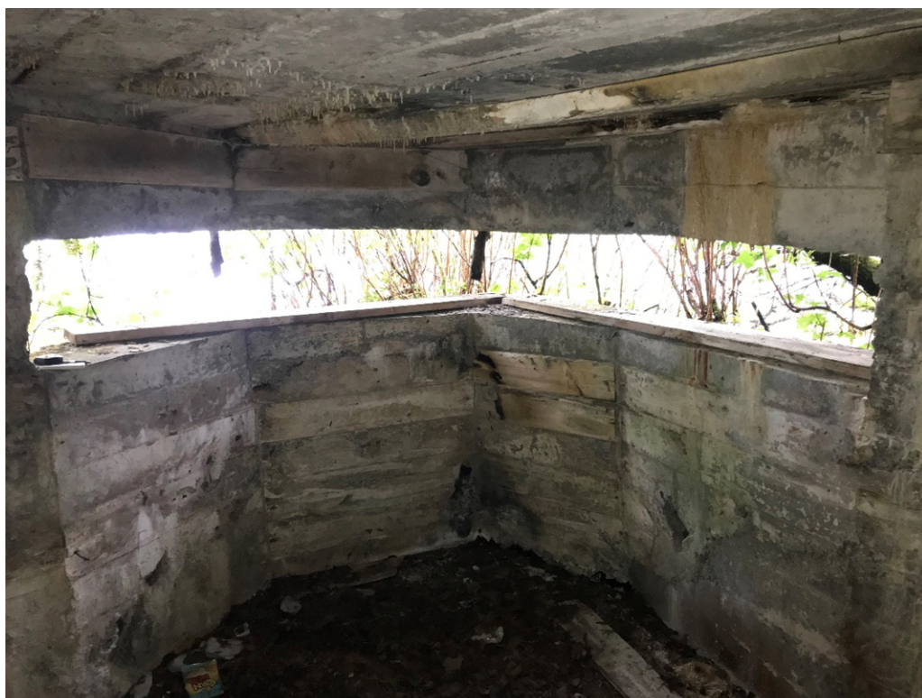
Photograph 2: Interior of Observation Post (May 2020)
